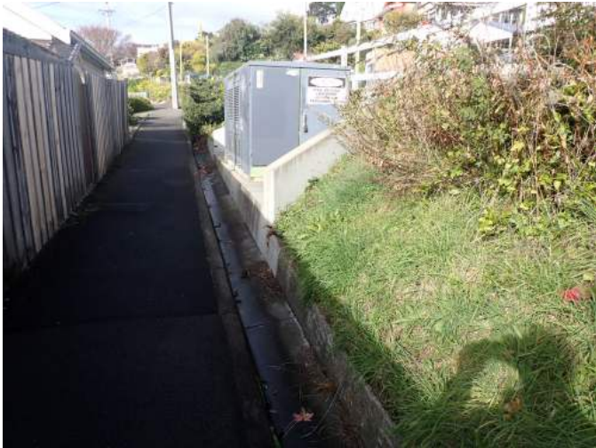
Plate 5. Main L. cylindracea site at Proctors Road, Dynnryne. Three specimens were found on the bare concrete wall in front of the electricity substation and one on the ground behind it.
