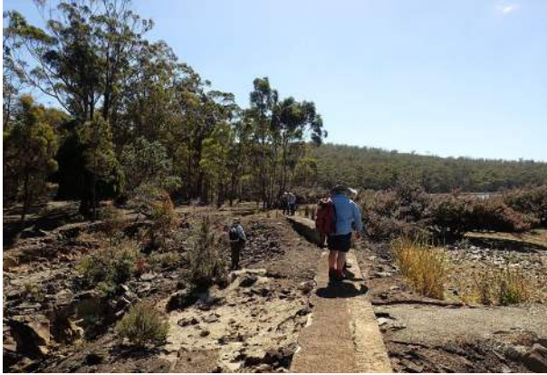
Plate 2: Walking along the dam wall
