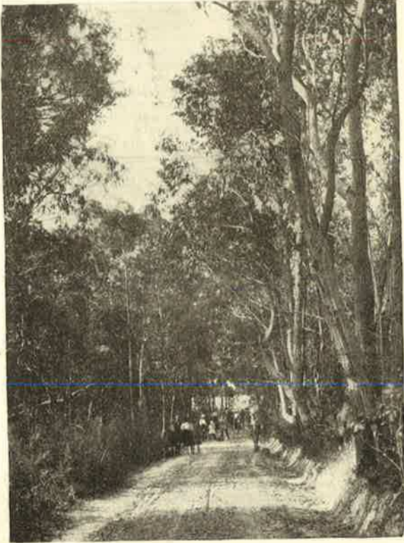
Safety Cove Road, Port Arthur.
